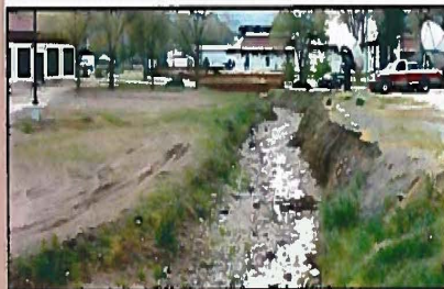
The current campus waterway
