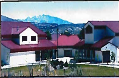
Front view of the solarium site
