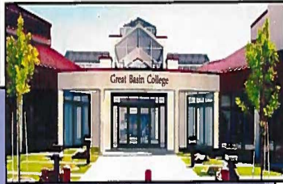
Front view of the solarium
